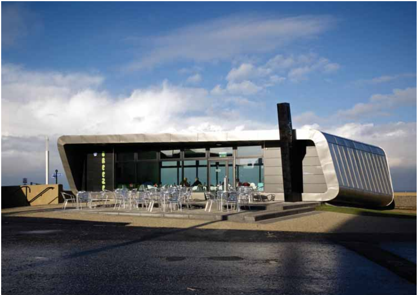
View of the sunny south elevation from the street, showing the silver 'ribbon' element framing the view.
