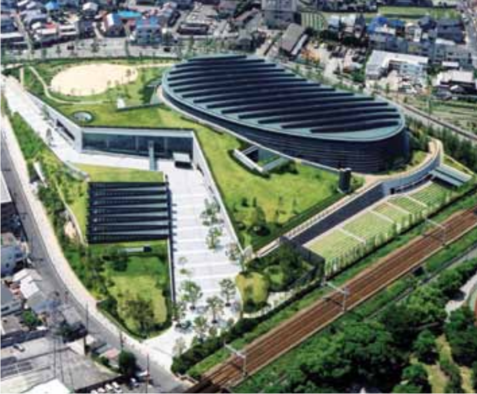
The Nishikyogoku Swimming Pool Complex is a seamless mix of earth and architecture.
